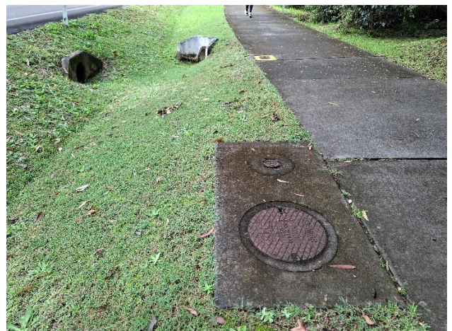
Plate 16: Sewer access and culverts
